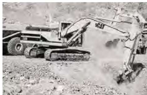
Gambar 6.4 Operasi dozer saat excavating dan loading
