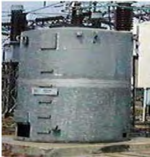
Gambar 5.8. Resistor Jenis Cairan ( liquid resistor )
