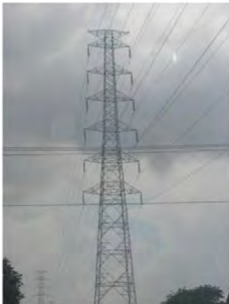
Gambar 4.8 Tower 4 sirkit tipe suspensi tipe tension
