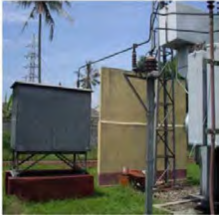
Gambar 5.6 Resistor Jenis Logam ( metallic resistor )
