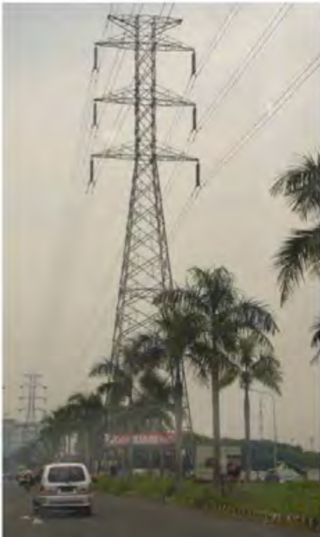
Gambar 4.10 Tower 2 sirkit tipe suspensi
