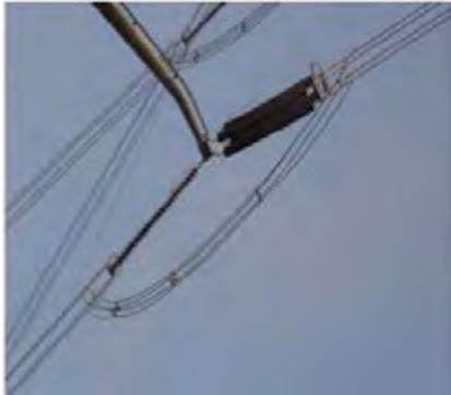
Gambar 4.33 . Tension clamp 5. Suspension clamp
