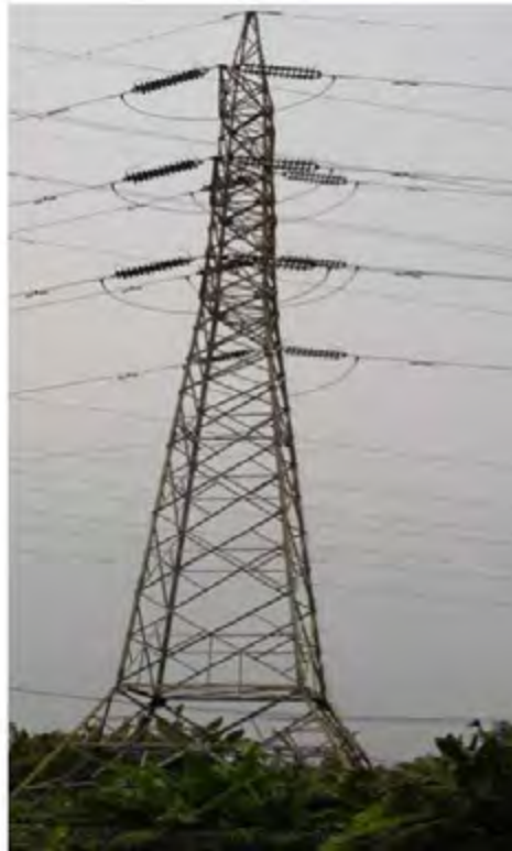
Gambar 4.11 Tower 2 sirkit tipe tension
