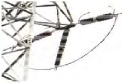
Gambar 4.32 Tension clamp
